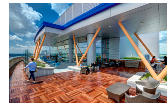
Cincinnati Children's Clinical Sciences Pavilion Rooftop Terrace Cincinnati, Oh Full Architectural Services
