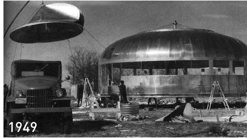
1949 Wichita House A Dymaxion prefabricated, single family dwelling unit designed by Buckminster Fuller.
