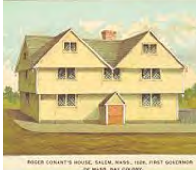
1624 Great House, Cape Ann The first known prefab, a panelized woodhouse, is shipped from England to Massachusetts as housing for a fishing fleet.
